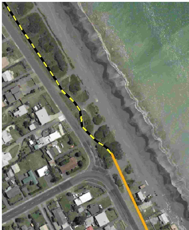
Major beautification is planned to correspond with the Beach Rd-Clifton Rd section of the cycleway
